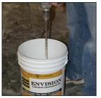
Mix Envison Concrete & Color with drill and mixing paddle.
